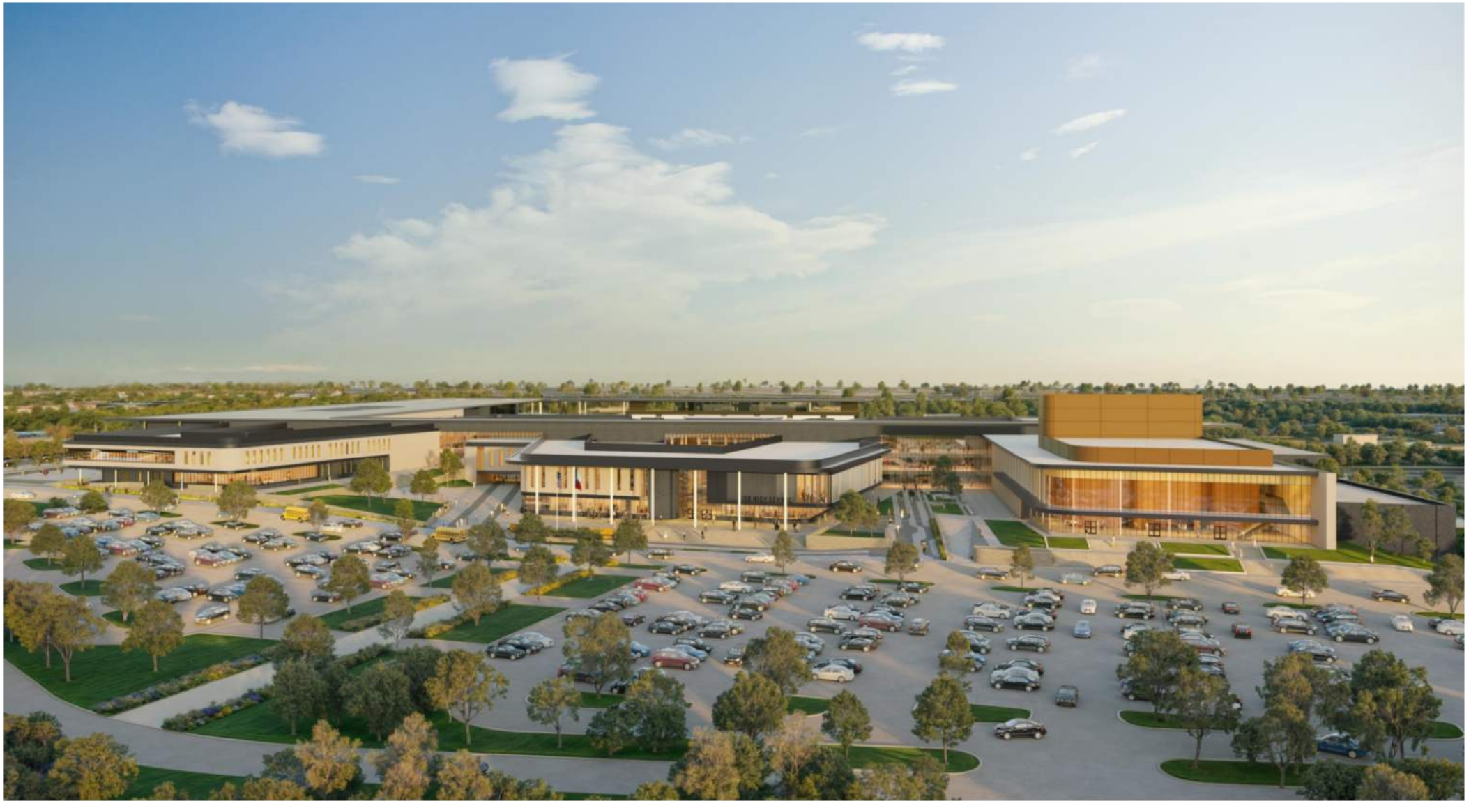
overall east side elevation
