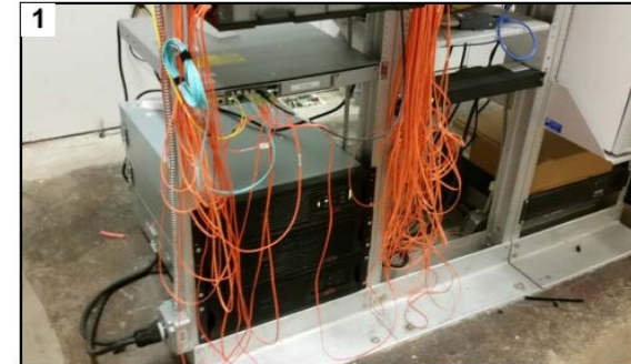
e. Clearances behind the equipment racks are limited and do not meet the NEC requirements for 36" of working clearances. The UPS constricts access to the rear working area of the rack.
