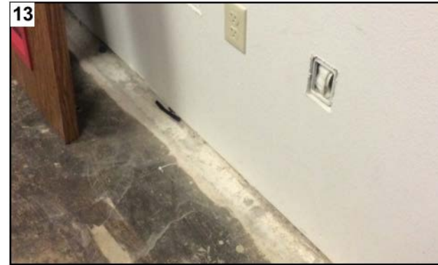
80% of the rubber base is missing.
