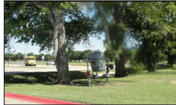
Add concrete bollards around gas meter.
