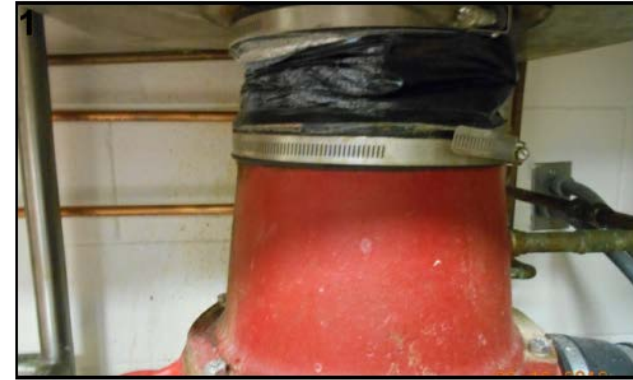
The connection of the disposer to the dish table is deteriorating.
