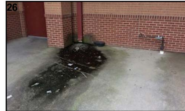
Roof shed water staining at the service bay gutter downspouts appear to have grease residue from the roof mounted vents.
